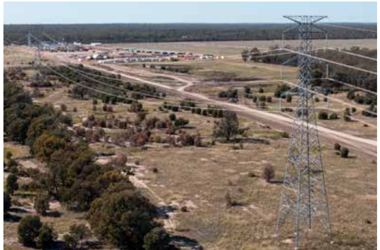
Western Downs Green Power Hub. Image Courtesy: Queensland Government
